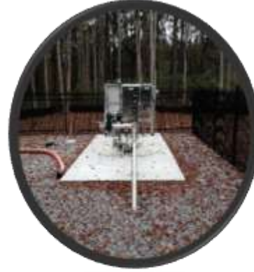
Sanitary Sewer Collection
